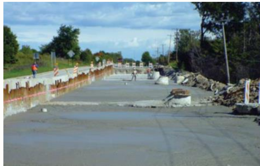
Central Road w Schaumburg w stanie Illinois (USA) [Short A., Kinniburgh W.: Lightweight concrete. Asia Publishing House, 1963]
